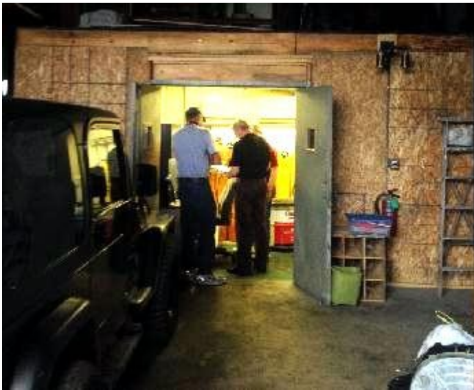
Dave, Mike, and ?Justin finishing up in the new comp room.
